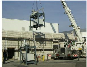
Figure 2: Linde TCF-50 Cold-box for 180 l/hr, 4.2-K LHe production (top), and Leybold vacuum pumps for 80-W, 1.8-K HoBiCaT operation being installed in the pump room (bottom).
